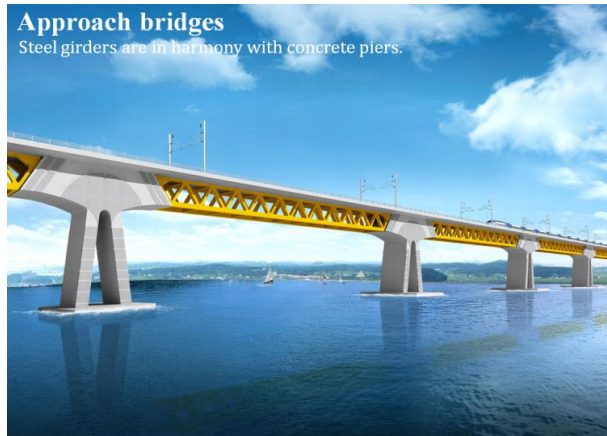
Fig. 26 Harmonized piers & girders in Seohae railway bridge.
