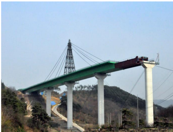
Fig. 7 Site view during launching.
