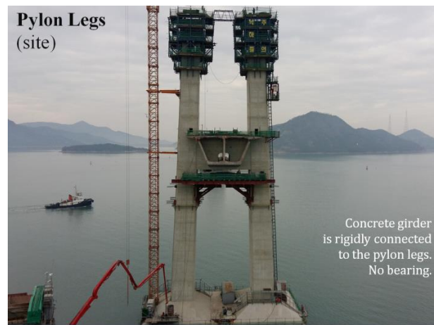
Fig. 19 Pylon during construction of Cheonsa bridge.
