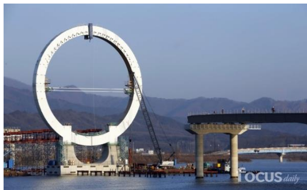
Fig. 14 View during construction of Chuncheon bridge.
