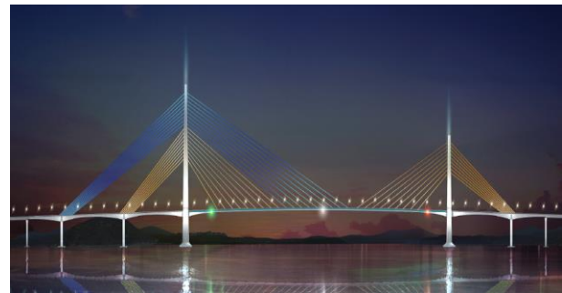
Fig. 18 Night view of Cheonsa bridge.
