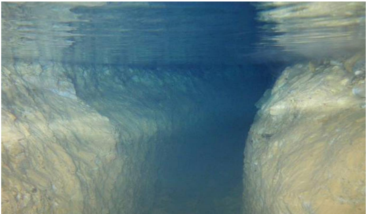
Fig. 8 An underground water channel documented within the Ravne tunnel system.
