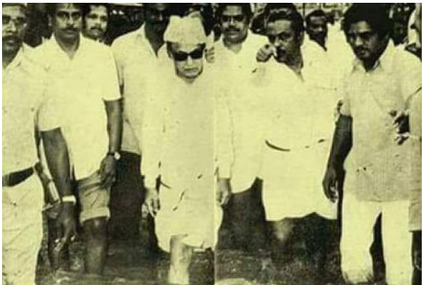
Fig. 5 Former Chief Minister, M.G. Ramachandran in knee-deep water during the 1985 floods [6].
