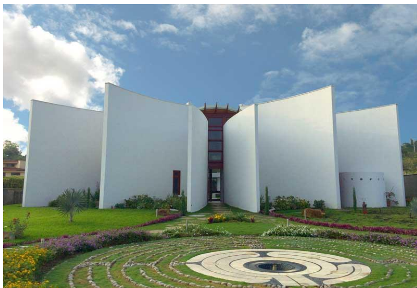
Fig. 1 Mariposa house. Cali. Colombia (Projected by Luis de Garrido). North façade.
