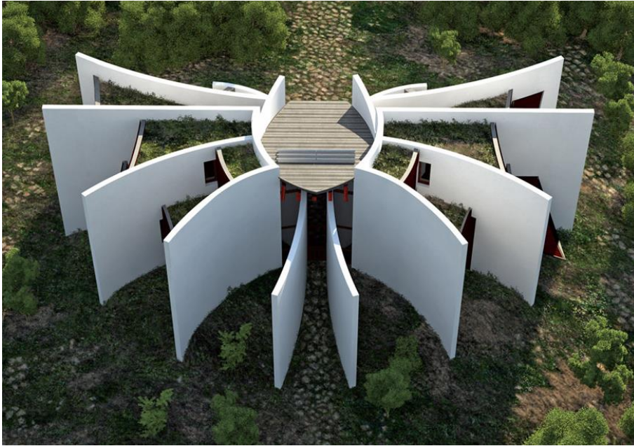
Fig. 4 The Mariposa house has two types of roofs. The green roof covers the ground and first floor spaces, while the central double-height space has a sloping roof. The special design of the sloping roof forces the heated air to rise and escape through the highest part of the north-facing windows. This extraction of hot air creates a suction current which, in turn, creates a current of cool air by extracting the cooled air in the basement.
