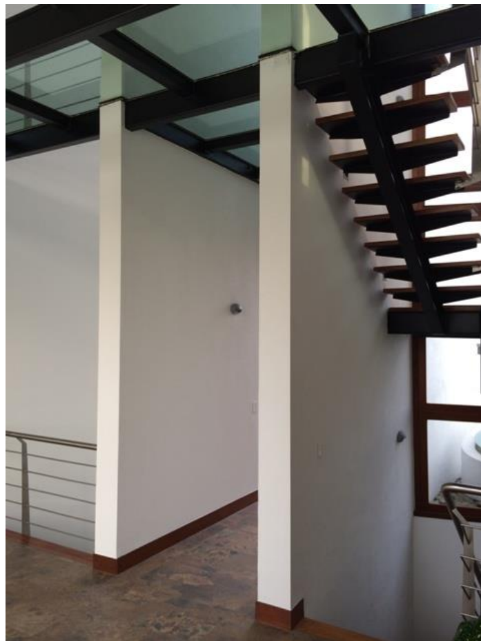
Fig. 13 Glass floors allow for greater lighting inside the house.
