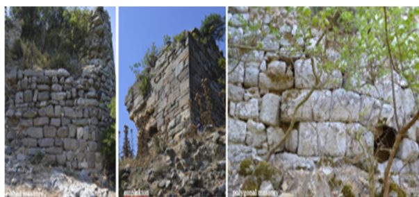
Fig. 2 Types of masonry walls.
