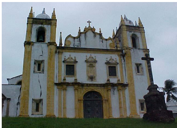
Fig. 3 Structural Damage in the Church of Carmo's in the middle of the year 2000.
