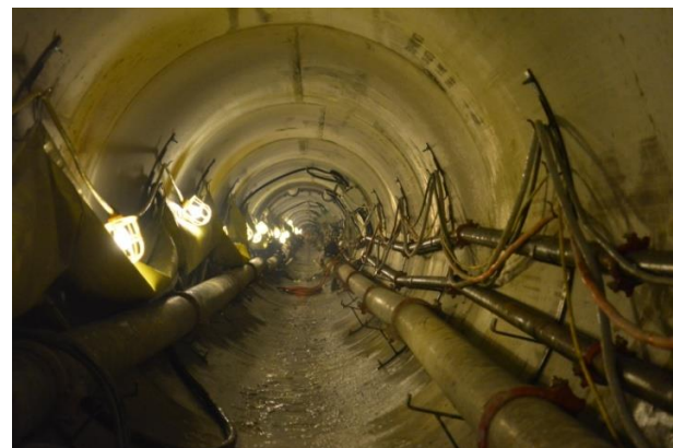
Fig. 2 View inside 1500mm ID Microtunnel - Elgin Mills.
