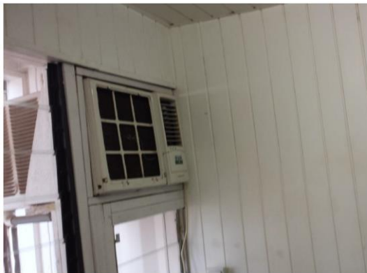
Fig. 7 Internal wall cladding and cooling system.
