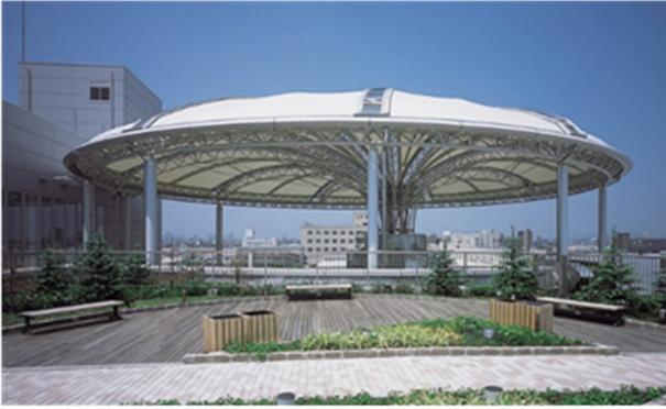
**Fig. 1** An example of domed free roof (provided by Taiyo Kogyo Corporation).
