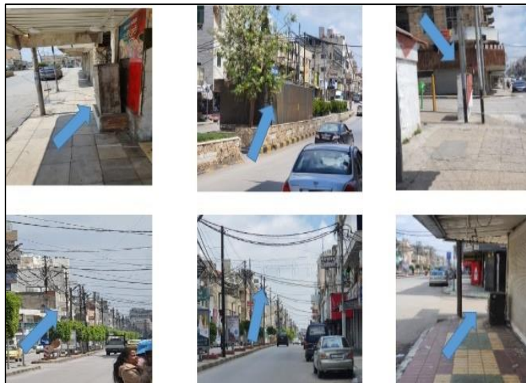
Fig. 2 Al-Hashemi street generators and electricity pole.
