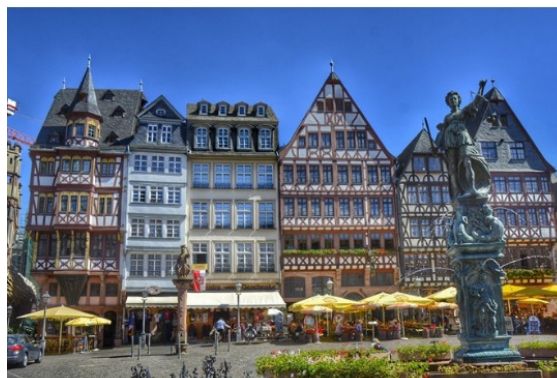
Fig. 3 Reconstructed (1981-1984) the eastern front of the square.
