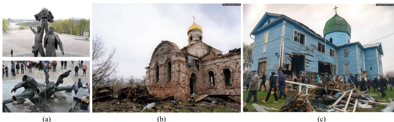
Fig. 12 (a) The Ukrainian and Russian worker monument in Kyiv, which was demolished last April; (b) Church with severe damage in Lukasifka; (c) Church of the Nativity of the Virgin Mary and the damage inflicted during war in the village of Peremoha.
