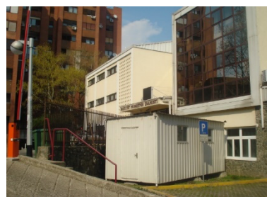
Fig. 2. Bicycle depot at Vukelićeva Street.
