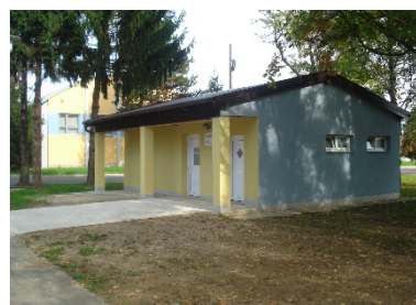
Fig. 1 Bicycle depot at Borongaj Campus.
