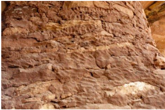
Fig. 4 A typical mud wall texture in Nigeria.
