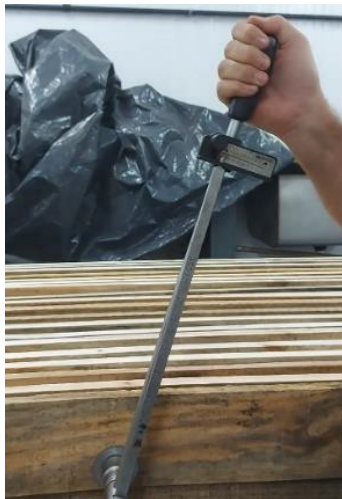
Fig. 9 Application of prestressing.
