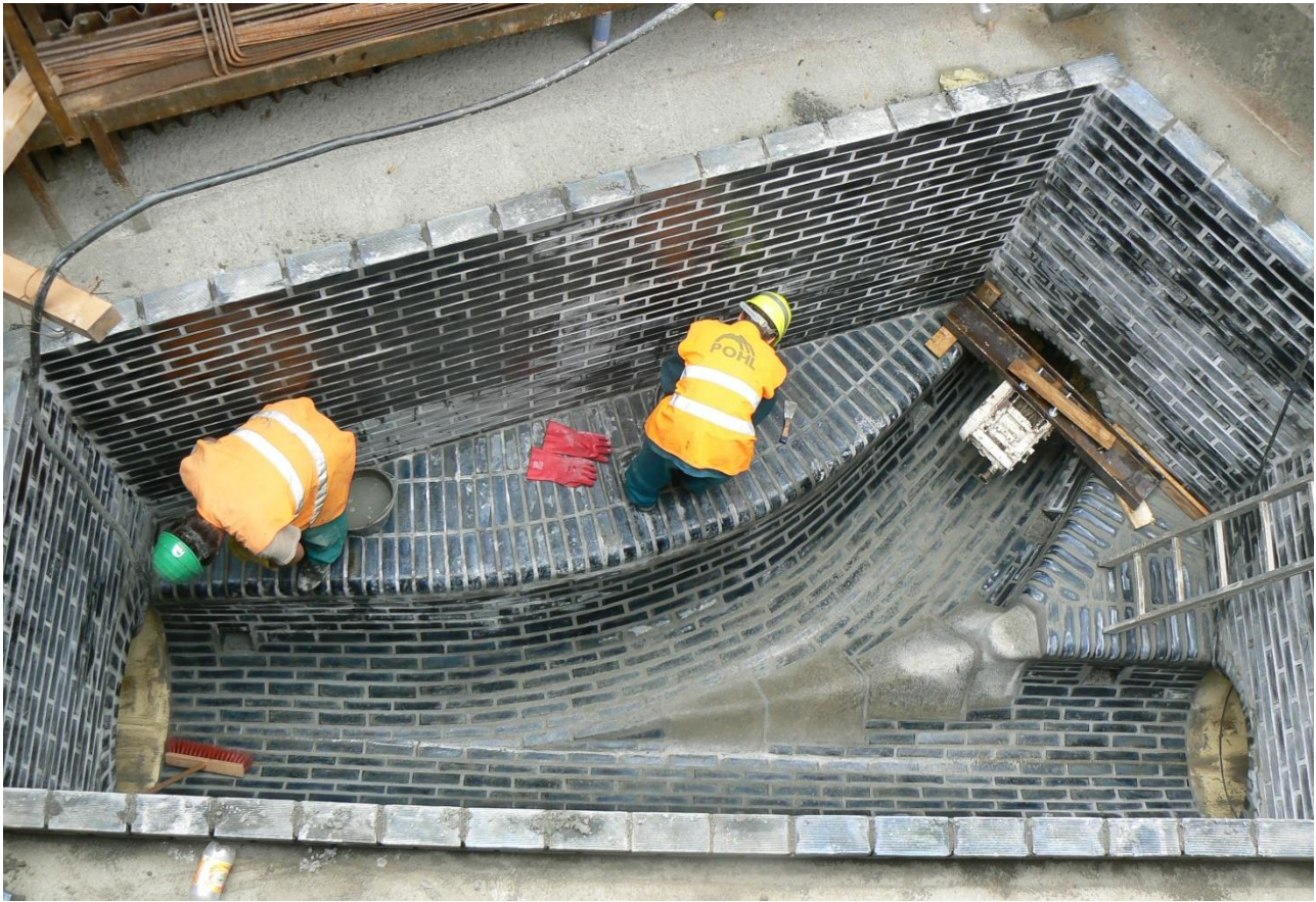
Fig. 6 Converging chamber of sewer (photo by Jan Mrzilek in 2011).
