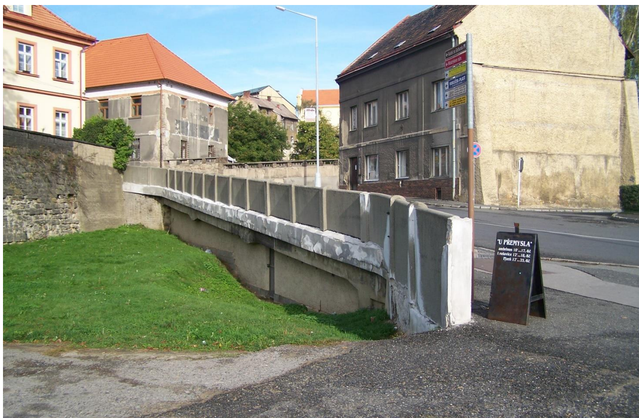
Fig. 1 Original concrete ramp as the main entrance to the historical centre of town Slany (photo by Jiri Novotny in 2006).
