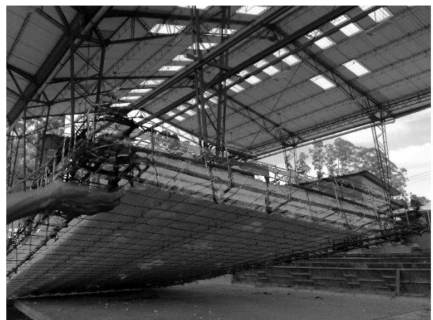
Fig. 5 Expanded polystyrene sheet with reinforcing steel.
