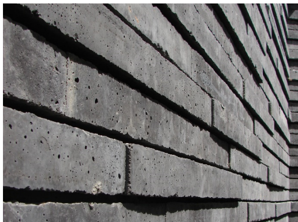
Fig. 8 Textured precast concrete elements to auto-shade.
