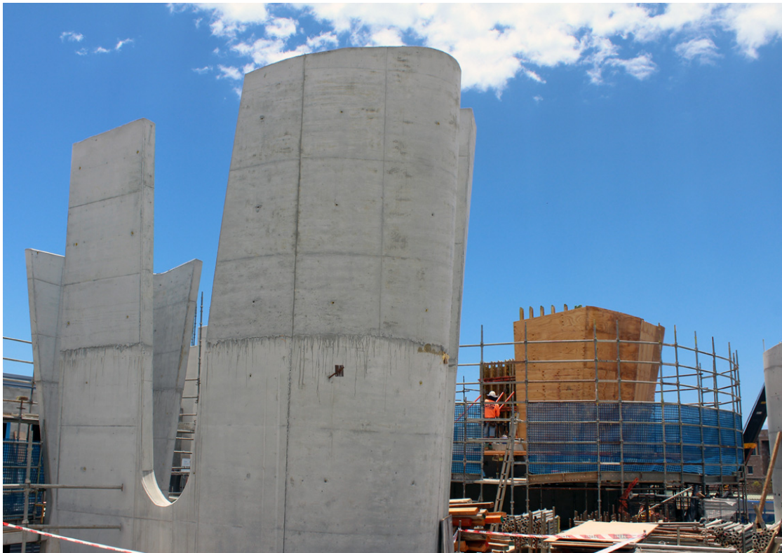
Fig. 10 Construction process on site (photo by author).
