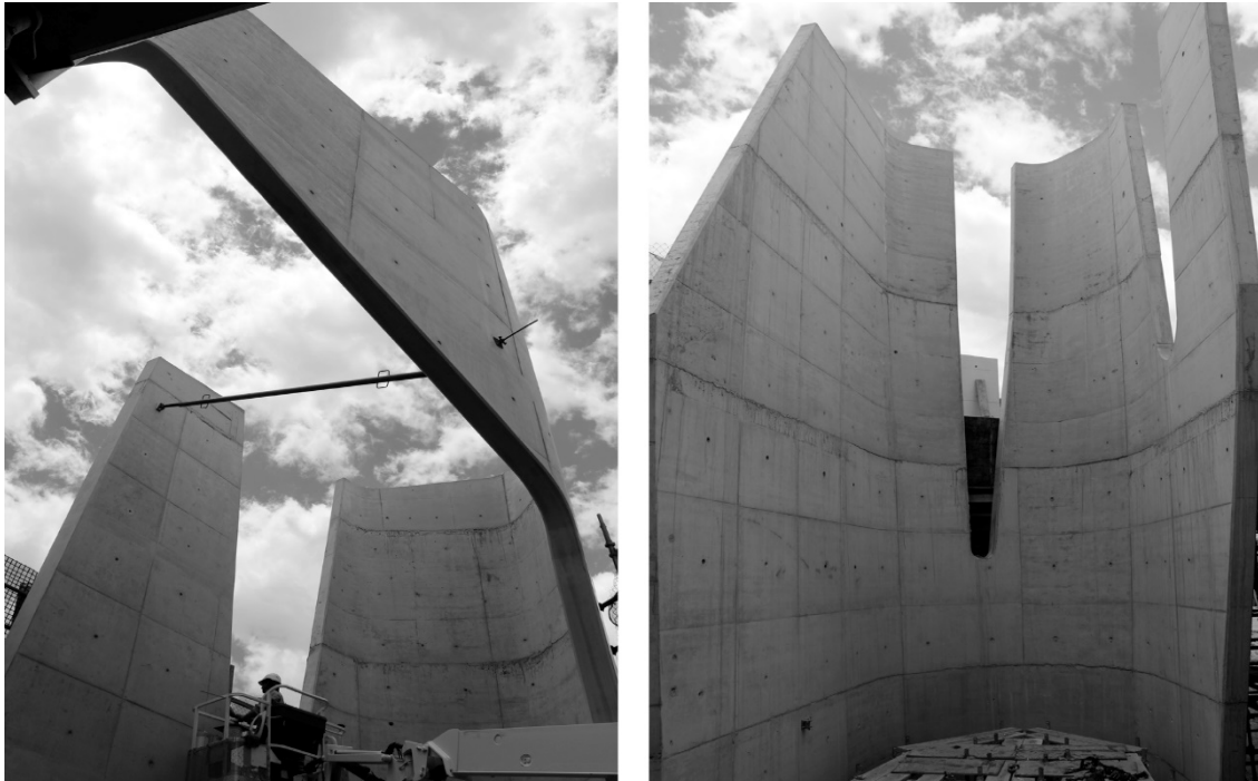
Fig. 11 “Scoops” nearing completion prior to roof placement (photos by author).
