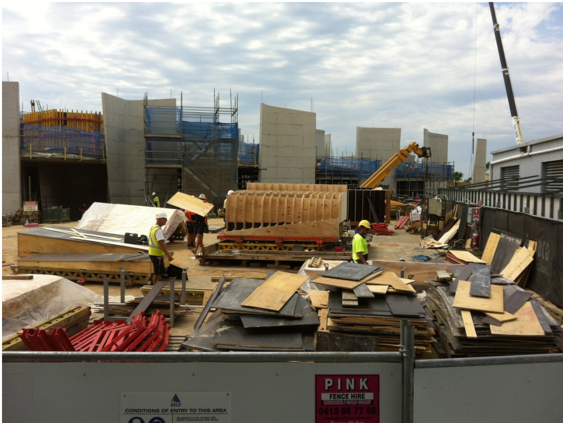
Fig. 9 Construction process on site—assembly area for formwork (photo by author).
