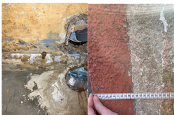
Fig. 5 Examples of sampling points for polychromy analysis.
