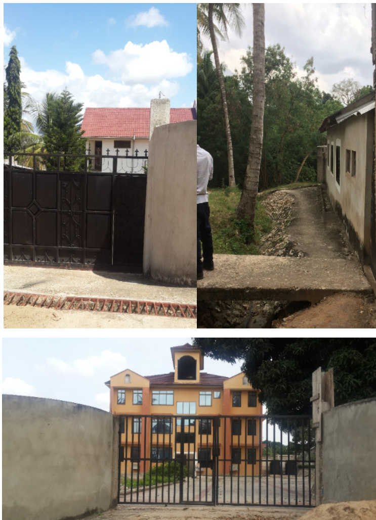
Fig. 21 Concreting and paving in the built areas.
