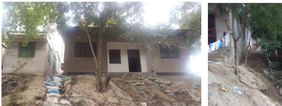
Fig. 20 Using sandbags to prevent erosion around buildings.
