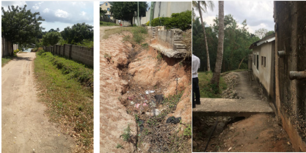
Fig. 17 Erosion along roadside due to cascading water field study in 2018.
