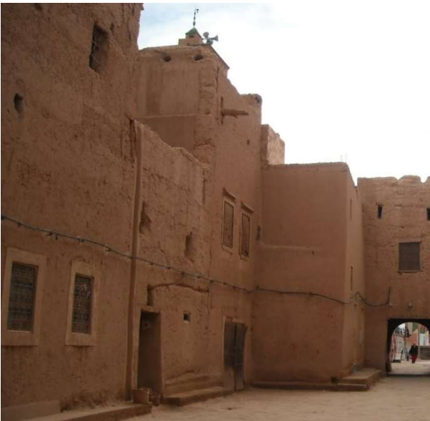
Fig. 3 The raw earth construction in Tinejdad oasis.
