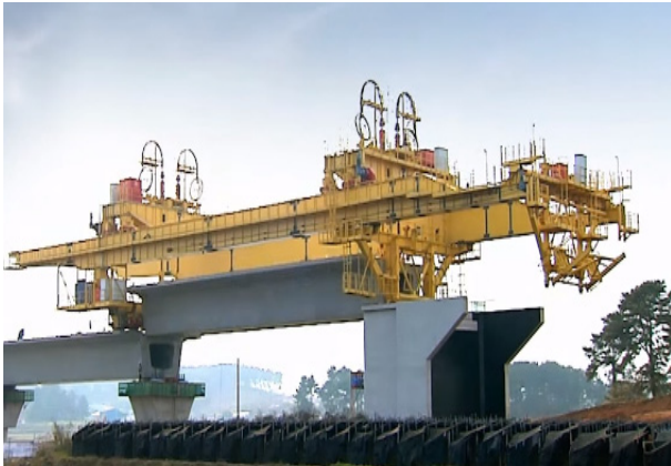
Fig. 1 Full span launching method.
