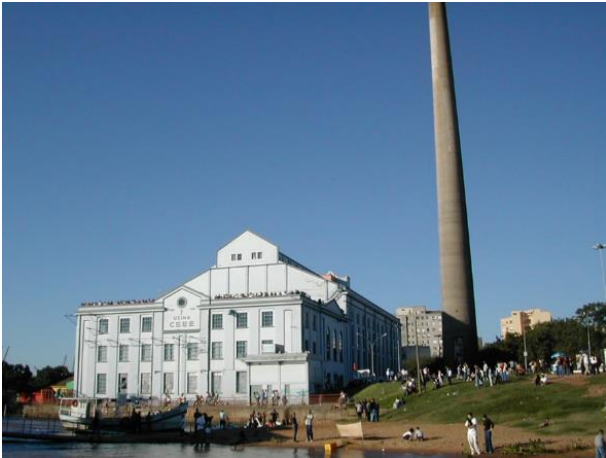
Fig. 1 The Gasometer Plant in Porto Alegre, Brazil.
