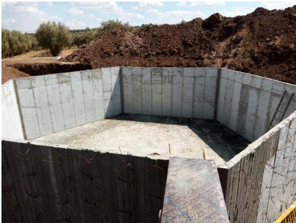
Fig. 3 Concrete box for nullifier.
