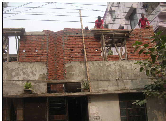
Fig. 5 Brick masonry at 1st floor after completion of ground floor.
