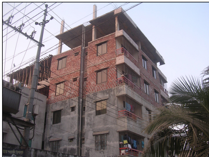
Fig. 8 Incremental addition of 3rd, 4th and half portion of 5th floor.
