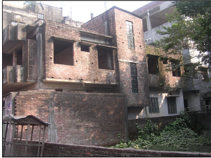
Fig. 6 Incomplete 1st floor (brick work & RC roof).
