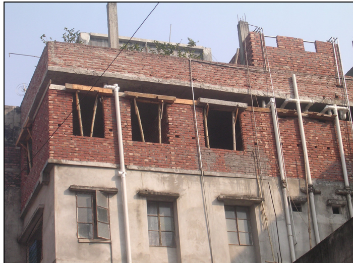
Fig. 7 Incremental addition to 2nd floor.
