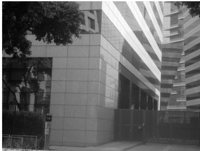
Fig. 8 The facades of Rochaverá Corporate Towers presents no stains. Source: Archive and photo of the author, 2017.
