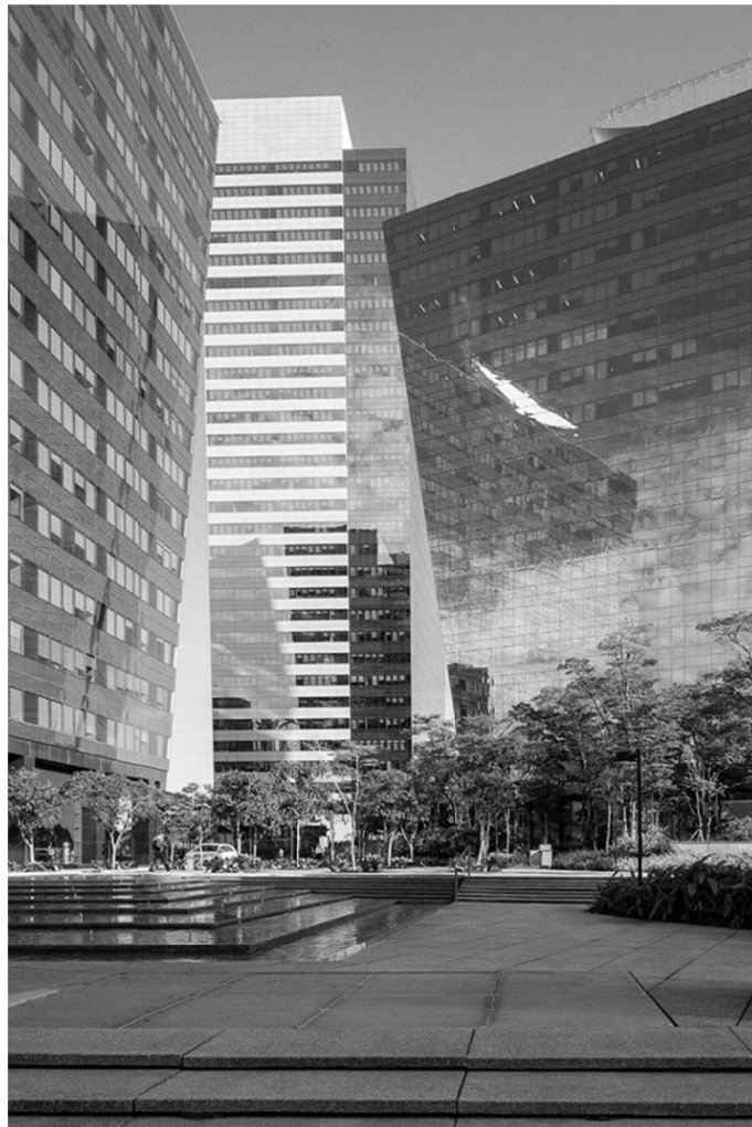
Fig. 6 Overview of the central square between the constructions and the access for cars [14].
