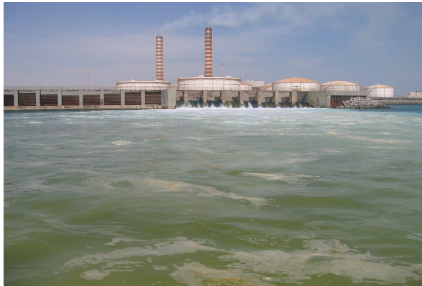
Fig. 2 Az-Zour desalination plant and outfall structure.
