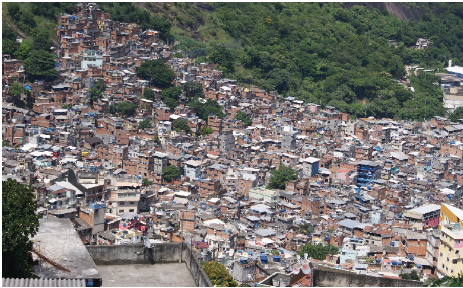
Fig. 3 A view from a higher position, the chaotic image of the buildings.
