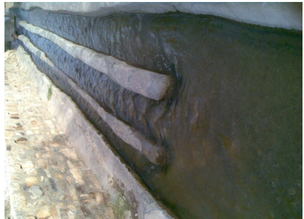
Fig. 3 Al-Khatmain splitting channel point, where as water coming from the main tunnel first divided into three equal parts, then one of the part remain along until reaching irrigated area while the two part joined into one channel, thus forming the two locally known Kiz; upper and lower.
