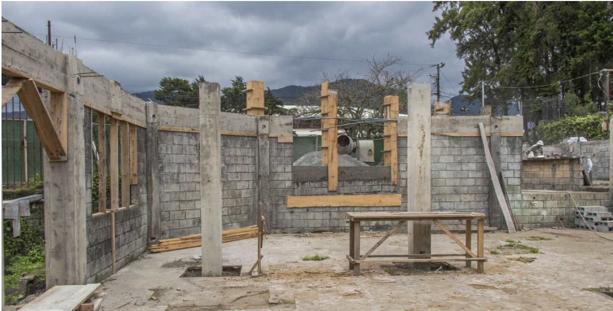
Fig. 5 Structural rehabilitation of existing damaged walls.
