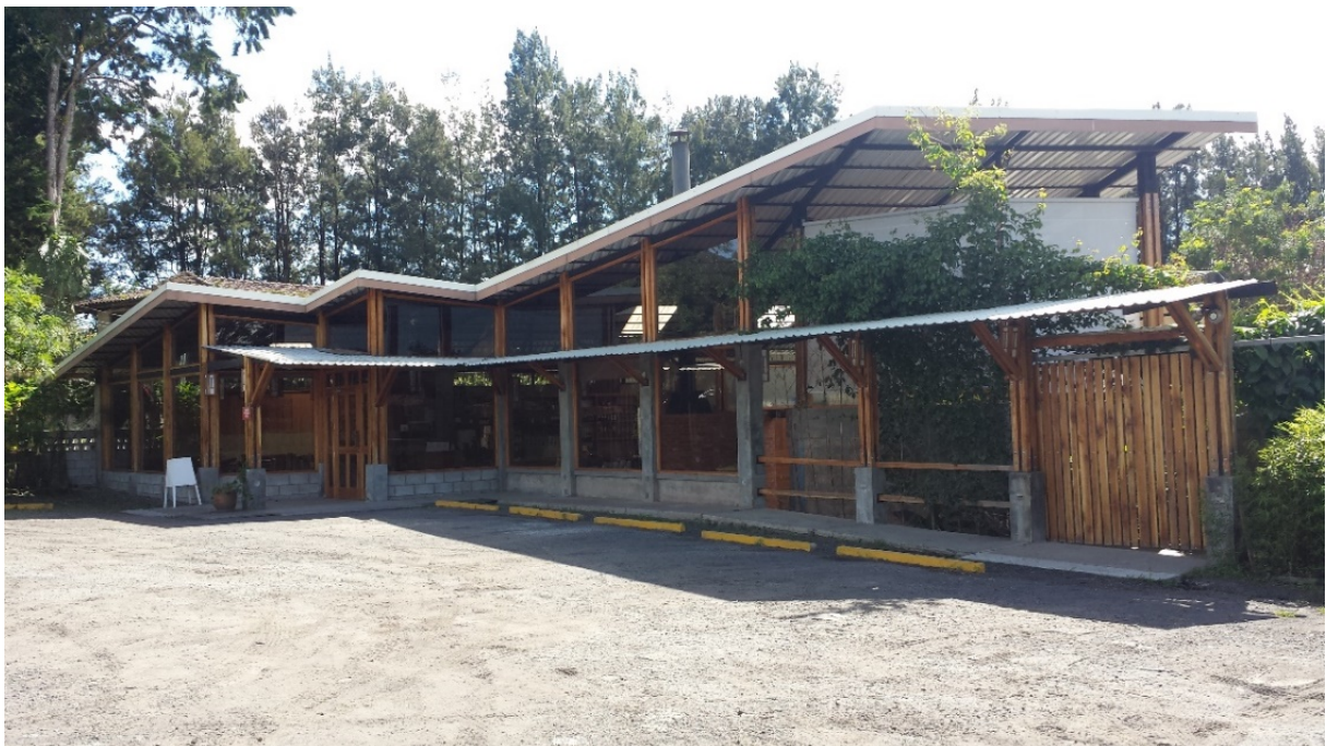
Fig. 8 Finished roadside café/restaurant.
