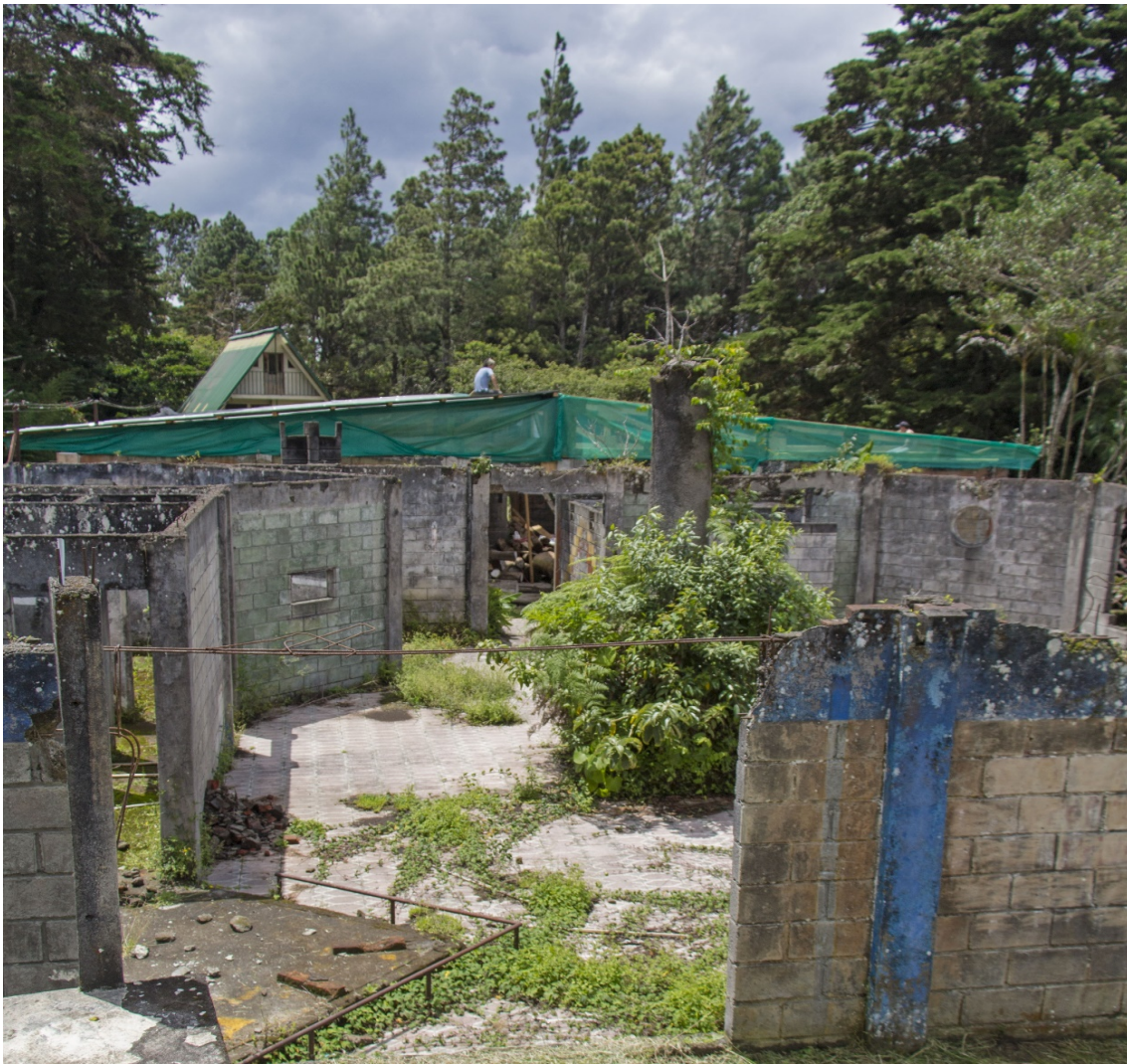
Fig. 4 Existing construction remains.
