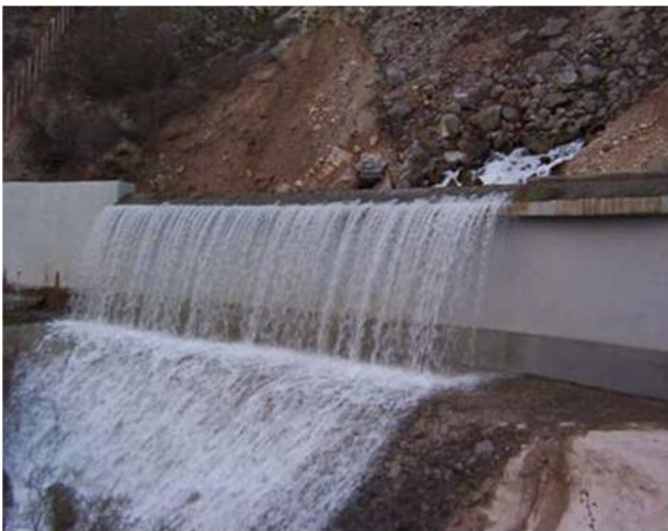
Fig. 3 Photo of dam in catchment facility.
