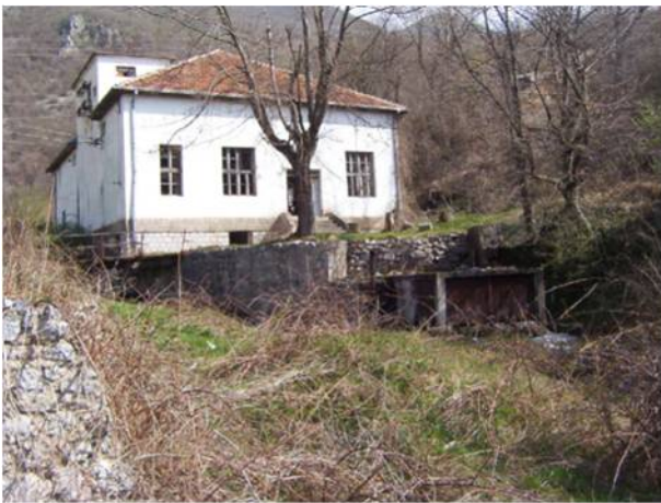
Fig. 8 Photo of hydropower building.
