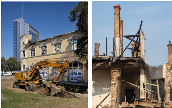
Fig. 4 The building was not professionally protected after the fire.
