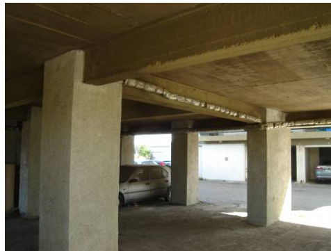
Fig. 25 Pyrgos Hardas building with columns at the ground floor “soft story” strengthened by R/C jacketing. The performance of this repaired building during the 2008 earthquake sequence was satisfactory without signs of any distress.
