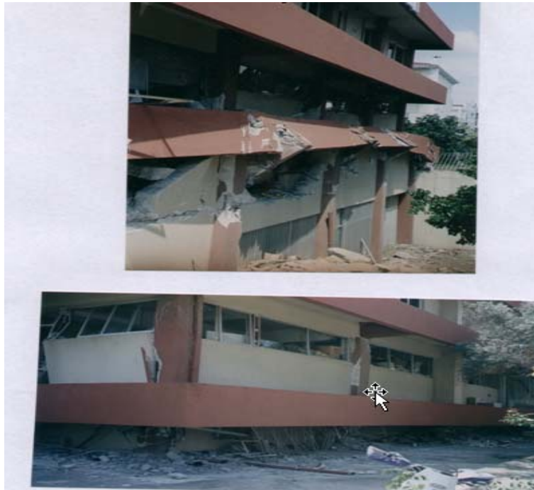
Fig. 20 Total collapse of ground floor with short columns—“Prokos” building (epicentral region).
