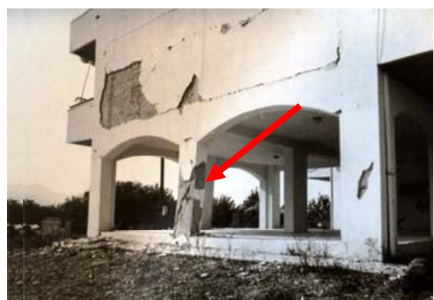
Fig. 5 (a) Damaged “soft story” in workers building (Kalamata); (b) Damaged “soft story”; (c) Damaged “soft story”.
