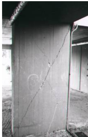
Fig. 26 Damaged column C35 of the Pyrgos Hardas Building.
