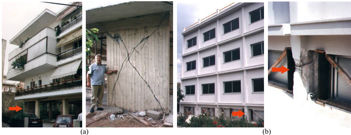
Fig. 11 (a) Damaged “soft story”; (b) Damaged “short” columns.
