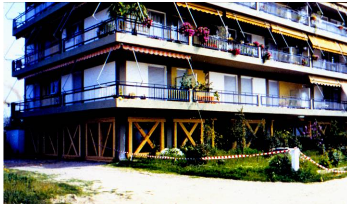
Fig. 24 Temporary strengthening of the damaged “soft story” of the “Pyrgos Hardas” building.
