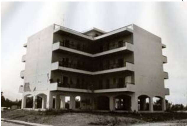
Fig. 5 (a) Damaged “soft story” in workers building (Kalamata); (b) Damaged “soft story”; (c) Damaged “soft story”.
