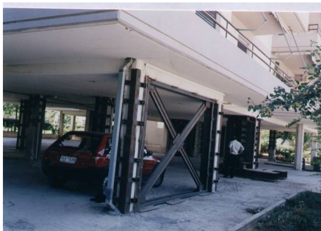
Fig. 18 Temporary strengthening of the damaged “Soft story” of the Metamorfosi building.
