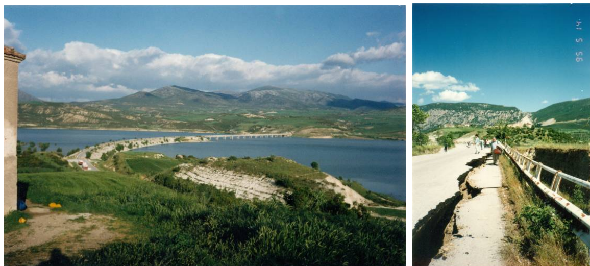
Fig. 10 Damaged abutment of the “Rymnio” bridge.
