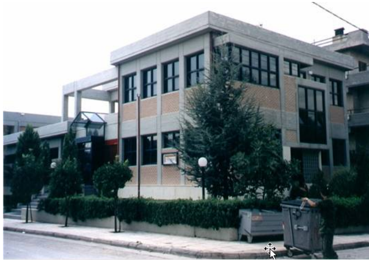
Fig. 19 Excellent performance of “Gnomon” building designed by the New Greek Seismic Code (epicentral region).
