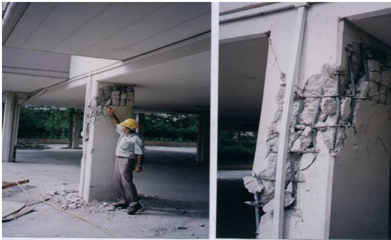
Fig. 17 Column shear failure – “Soft story” Metamorfosi building.
