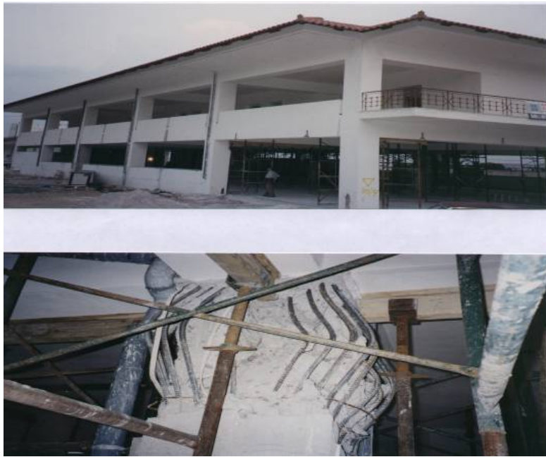
Fig. 16 Failure of all the central columns (epicentral region).
