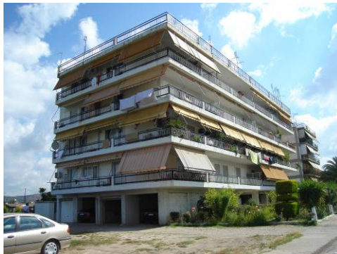
Fig. 25 Pyrgos Hardas building with columns at the ground floor “soft story” strengthened by R/C jacketing. The performance of this repaired building during the 2008 earthquake sequence was satisfactory without signs of any distress.
