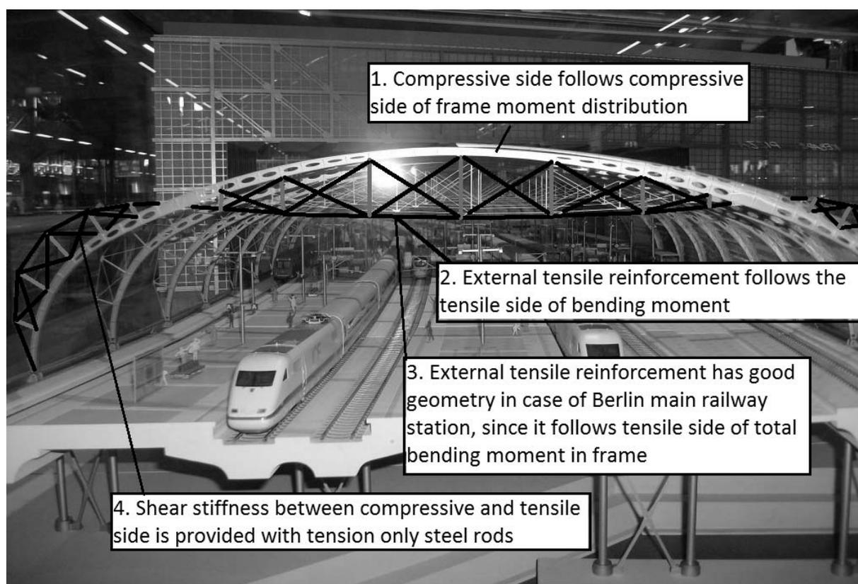
Fig. 6 Berlin Main Railway Tensile, compressive and shear struts arrangement.
