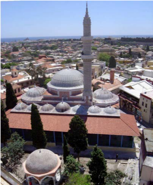
Fig. 3 The restored Suleiman mosque.
