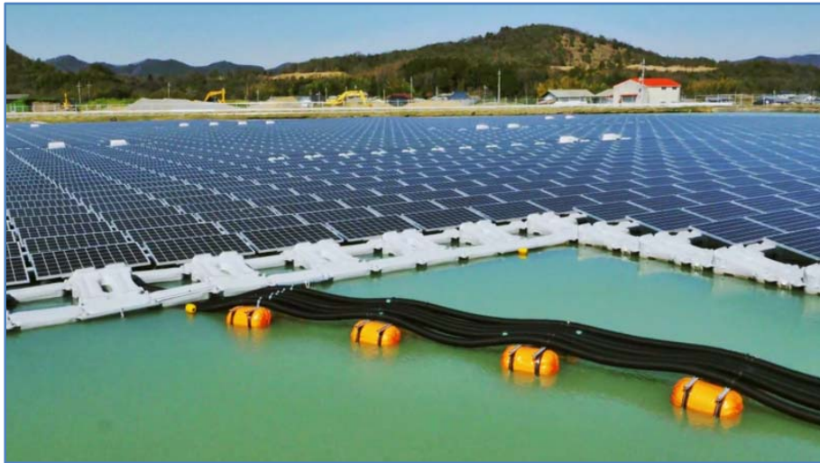
Fig. 1 Floating PV system in Hyogo—Japan (Source: Ref. [2]).
