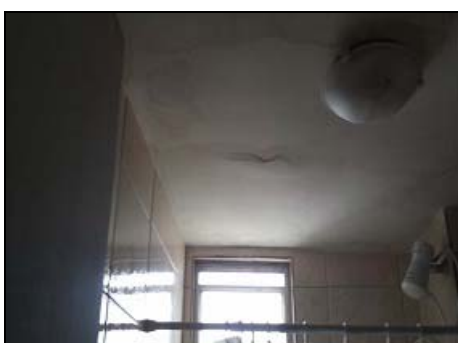
Fig. 4 Damage on the bathroom ceiling painting plaster.
