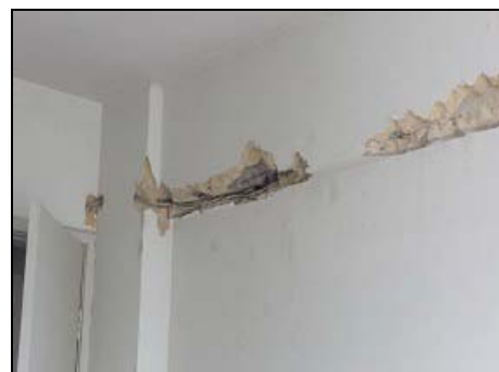
Fig. 5 Inspection of the electrical wiring (the repair must be done with ratio of 1:1:6 cement lime and sand mortar).
