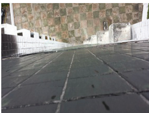
Fig. 13 The exposure to high temperatures damaged the adhesion between the ceramic plate and its substrate.
