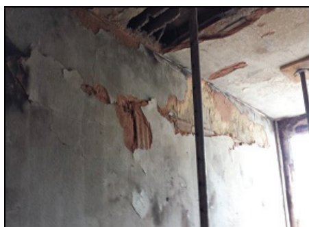
Fig. 9 Damage to the wall and the slab concrete block.
