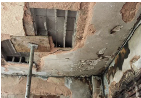
Fig. 12 Damage mortar and clay coating.
