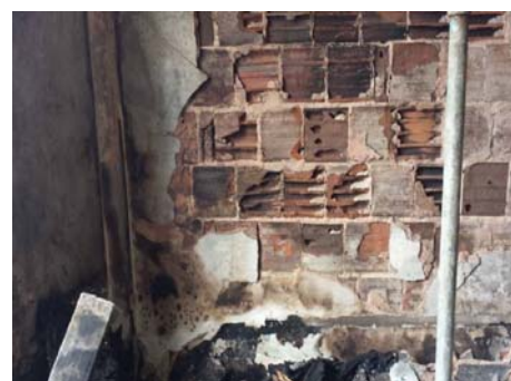
Fig. 7 Bedroom wall: damage to the plaster and coating mortar.
