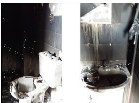
Fig. 17 Details of the damages of the sanitary ware.
