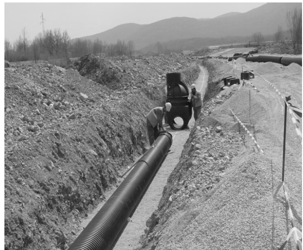
Fig. 7 Application of PEHD pipe system in drainage works [11].
