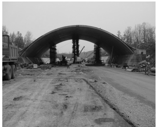
Fig. 8 Passage-bridge construction for the passage of wild animals [11].
