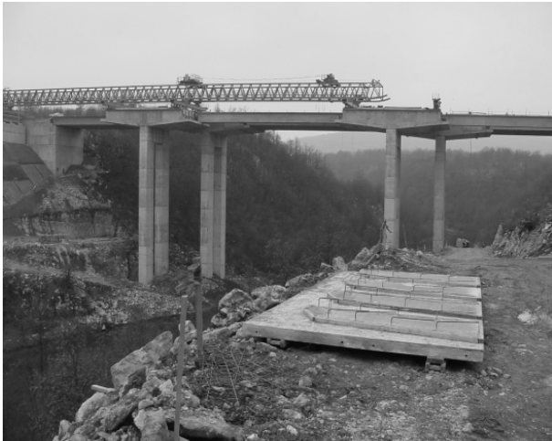
Fig. 6 Hammer beam application on the bridge [11].
