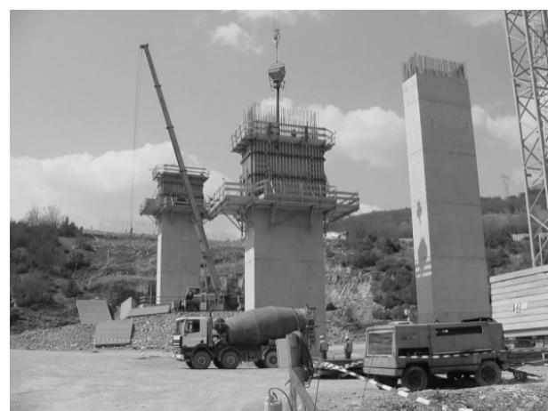
Fig. 5 Usage of climbing form in construction of viaduct feet [11].
