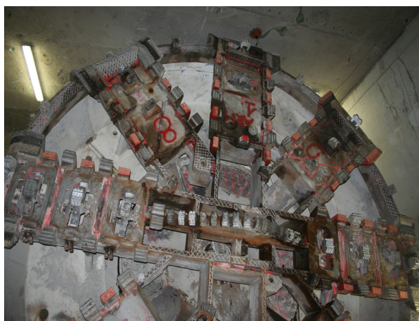
Fig. 8 TBM break-in from the Lotto station.
