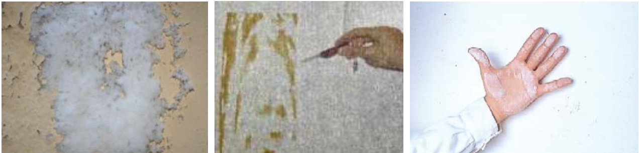
Fig. 8 Anomalies in painted walls.
