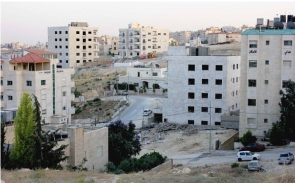
Fig. 9 Current practices of building on slopes in a north Ammani neighborhood.
