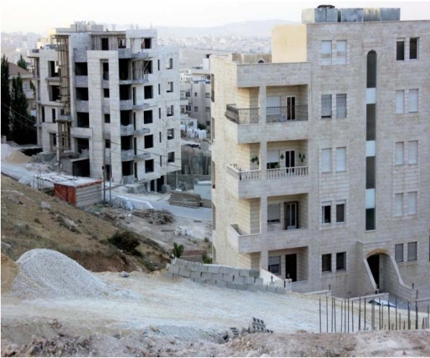
Fig. 6 Apartment buildings construction boom in Amman.
