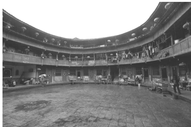
(b) Shared corridors of the whole buildings, Shanqing Lou in Chuxi Cluster
