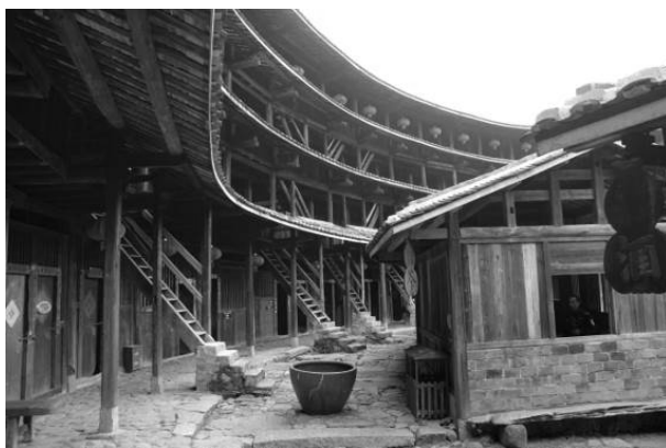
(a) Separate entrances and stairs for each family, Yuqing Lou in Chuxi Cluster
