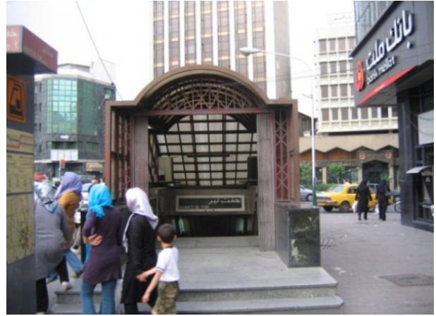
Fig. 4 Poor design of the station entrance.
