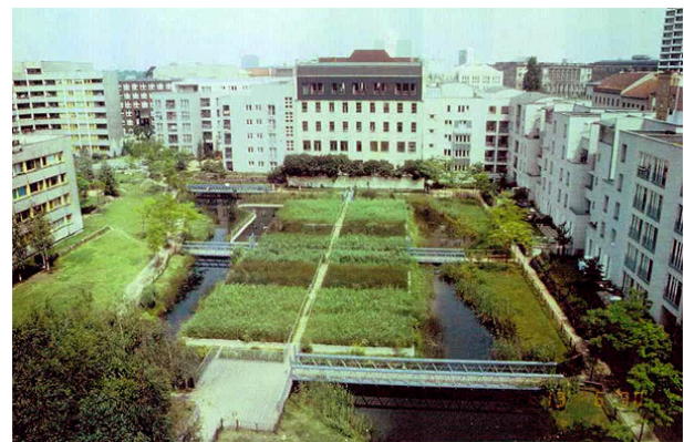
Fig. 12 Block 6 in Berlin. All wastewater from the households is purified in the courtyard of the settlement.
