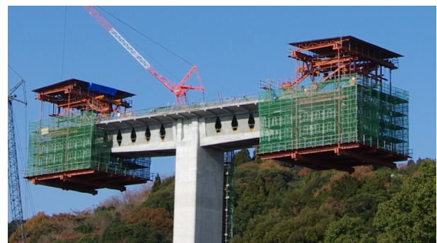
Fig. 7 Cantilever construction.
