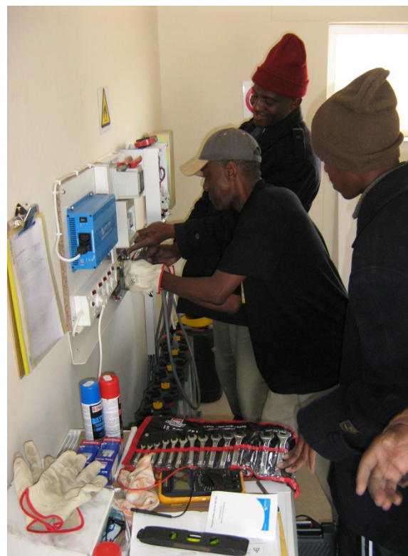
Fig. 4 Installation of interface equipment: battery system, inverter unit and metering units.
