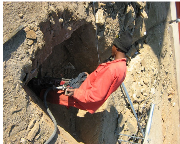
Fig. 2 Community member carrying out earth works for the wind turbine tower installation.
