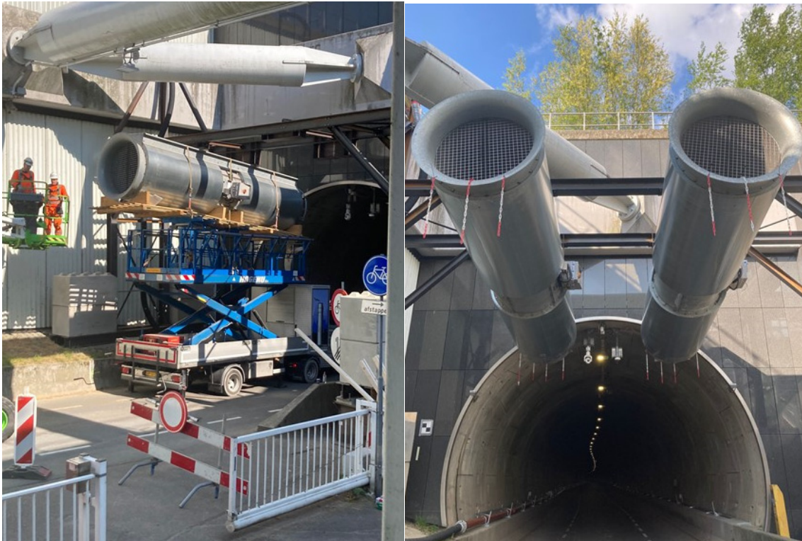
Fig. 9 In May 2022, the temporary extra jet fans to support public transport (busses) through the Second Heinenoord Tunnel are being mounted (pictures by Robin Witkamp, RWS).
