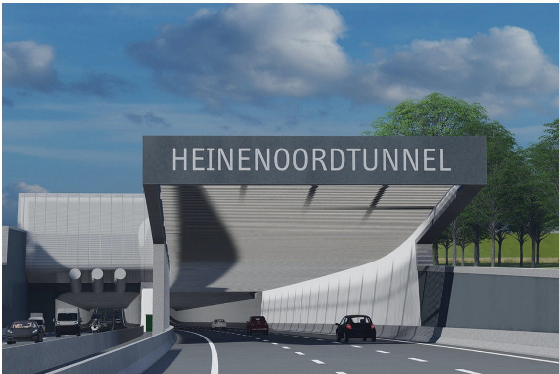
Fig. 7 Artist impression of the Heinenoord Tunnel after the refurbishment (Syb van Breda & Co Architects), view of the south portal; the green door between the tubes is one of the two exits of the escape gallery (the other one is at the north portal).
