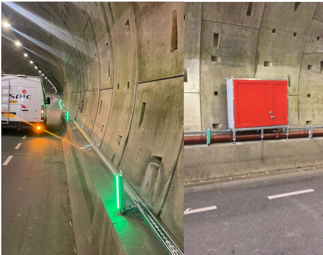
Fig. 10 In May 2022, the temporary evacuation lighting and fire extinguishing installation to support public transport (busses) through the Second Heinenoord Tunnel are being mounted (pictures by Robin Witkamp, RWS).
