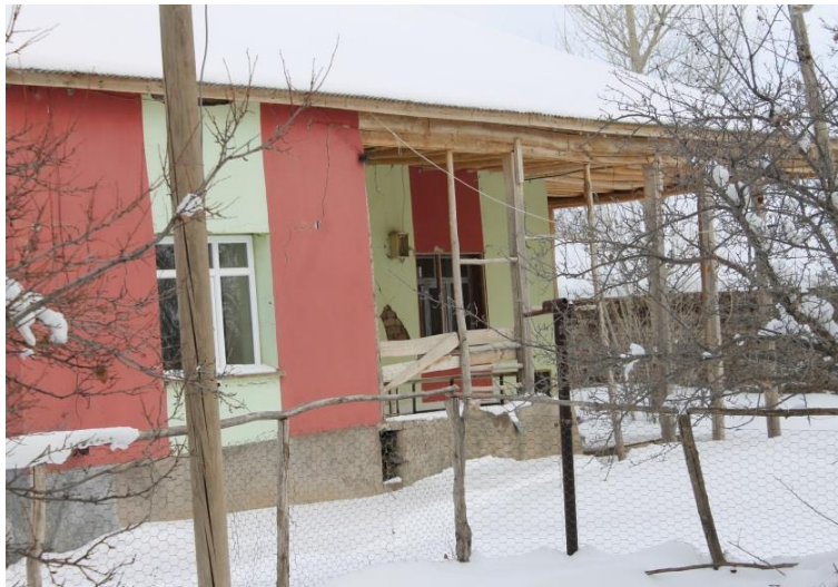
Fig. 15 Inhabited and maintained mud-brick building which is approximately 100 years-old (Esenpınar Village).
