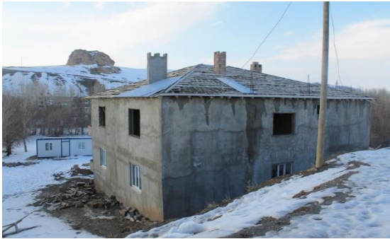
Fig. 8 Usage of bricks instead of mud-bricks (Bağdaşan Village).
