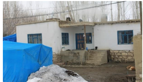
Fig. 13 A mud-brick building whose sub-basement elevation is sufficient (Kaymaklı Village).
