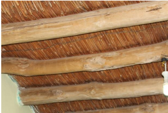
Fig. 7 Soil roof covering on old Van house (Esenpınar Village).
