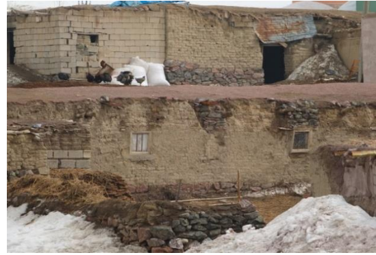
Fig. 10 The damages caused by the heavy and neglected roof covering (Dibekli village).
