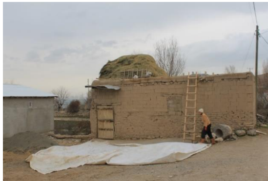
Fig. 12 Damages caused by usage of mud-bricks and bricks' being used together (Yeşilsu Village).
