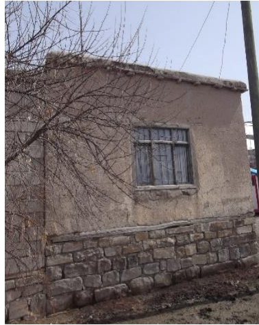
Fig. 14 A mud-brick building where horizontal joists were used in decently (Çalımlı Village).
