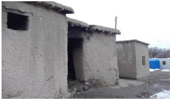
Fig. 9 Mud-brick buildings whose sub-basement elevation is not enough (Adıgüzel Village).
