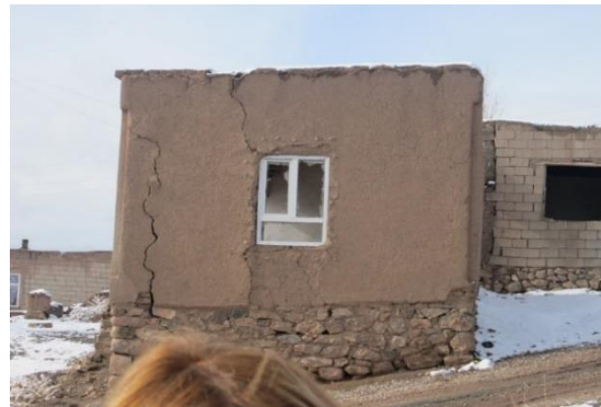
Fig. 11 Damages on the mud-brick buildings whose horizontal joists are non-existing (Ilıkaynak Village).
