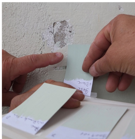
Fig. 5 Stratigraphic survey and essay of painting for the façade of the Petite Villa, 2012 © FLC.
