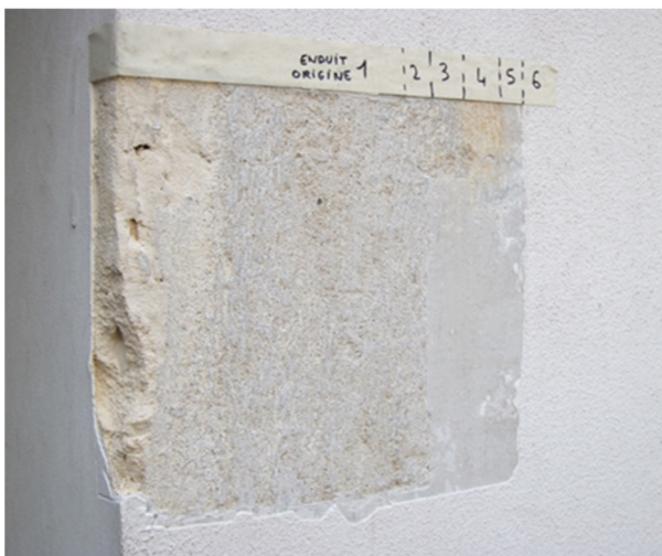
Fig. 4 Stratigraphic survey on the facade of the Maison La Roche: in layer 1 the original plaster (Cimentaline).
