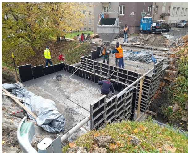
Fig. 6 Casting UHPFRC over-lays; transverse ties between wingwalls are also visible.
