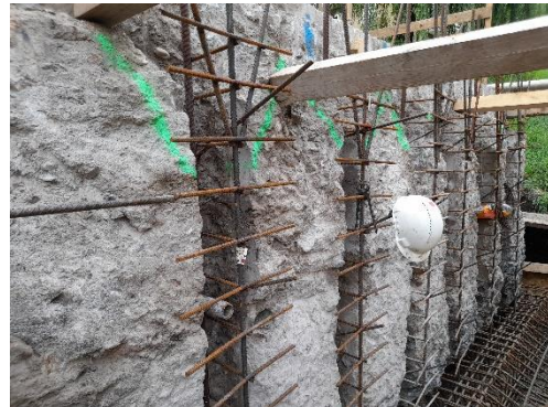
Fig. 4 Face of abutment with removed degraded concrete, gaps prepared for ribs and their reinforcement.
