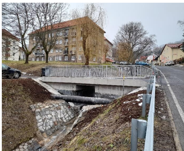
Fig. 7 View of the bridge after reconstruction; calculations proved that hydraulic capacity is sufficient even with the gas pipeline in front of the bridge.
