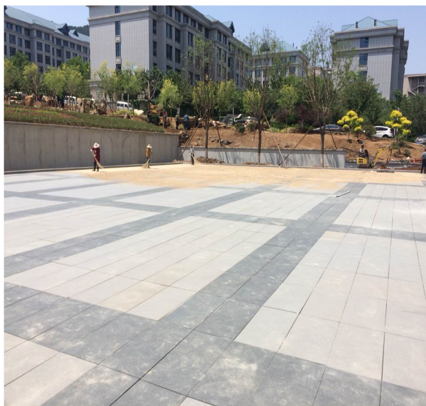
Fig. 2 Sand-based paver—typical field installation.
